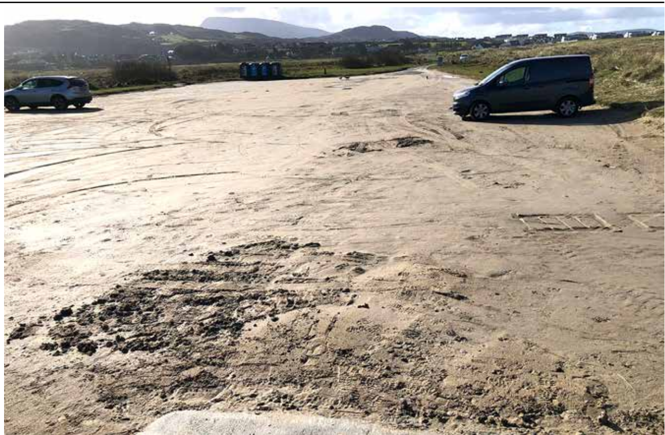
The effects of the recent storms as the sand covers the Car Park at Killyhoey Beach, Dunfanaghy
