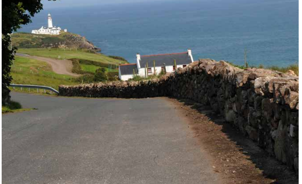
The finished wall at Araheera with the majestic lighthouse in the background.
