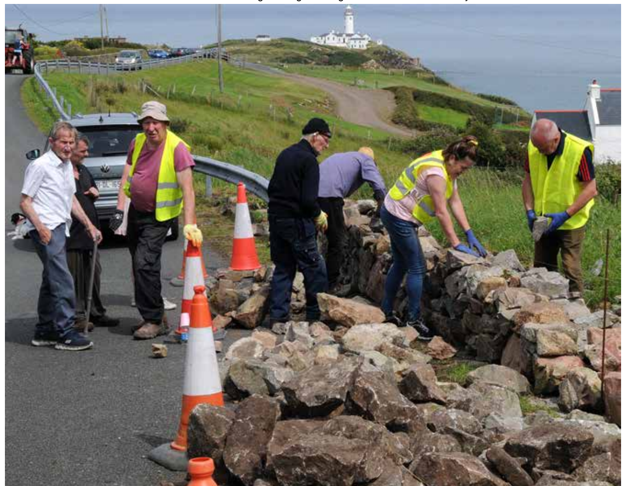
Jimmy Sweeney (with black cap) watching the construction of the wall.
