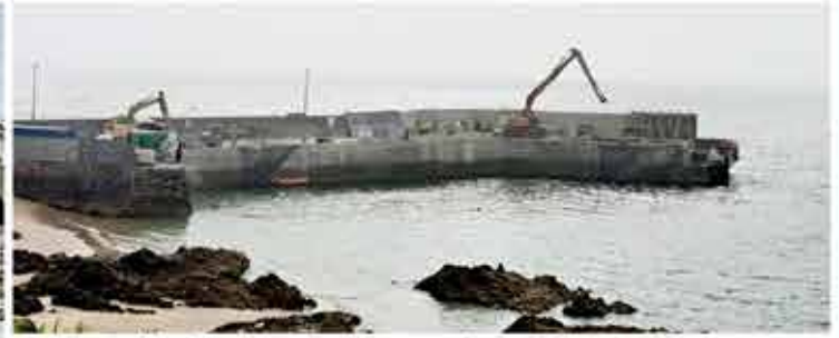
Work and renovations ongoing at Portsalon Pier
