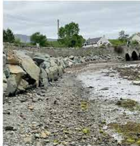
Rocks Armour at Ray Bridge
