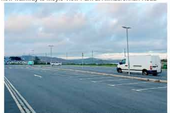
Newly renovated car park at Portsalon
