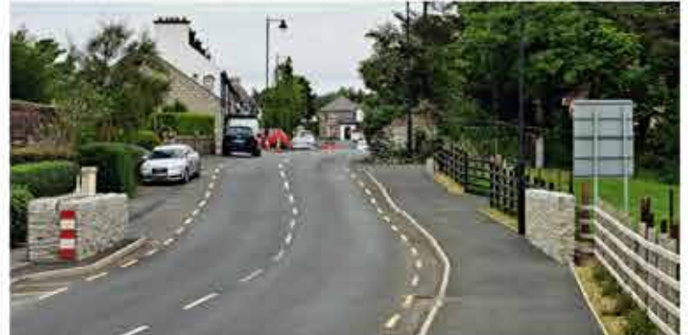
New bridge and footpath in Carrigart Main Street.
