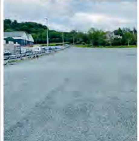
The resurfaced Car Park at the Milford Livestock Mart.
