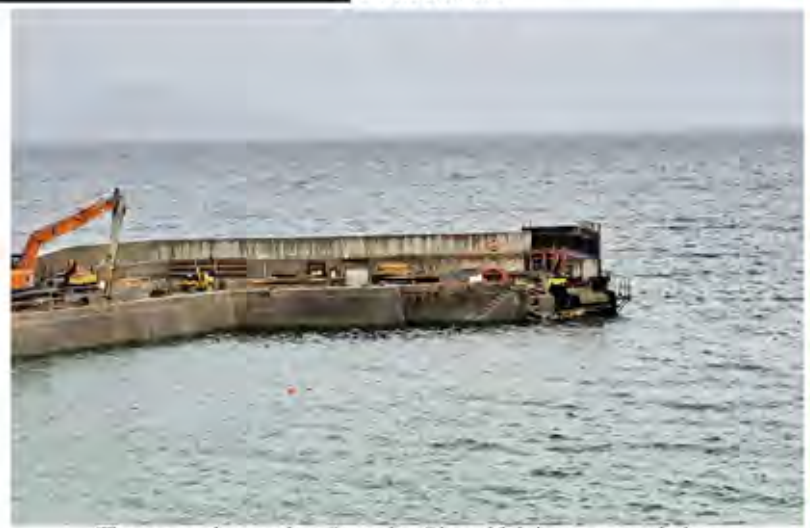
The renovation work at Portsalon Pier which is near completion.
