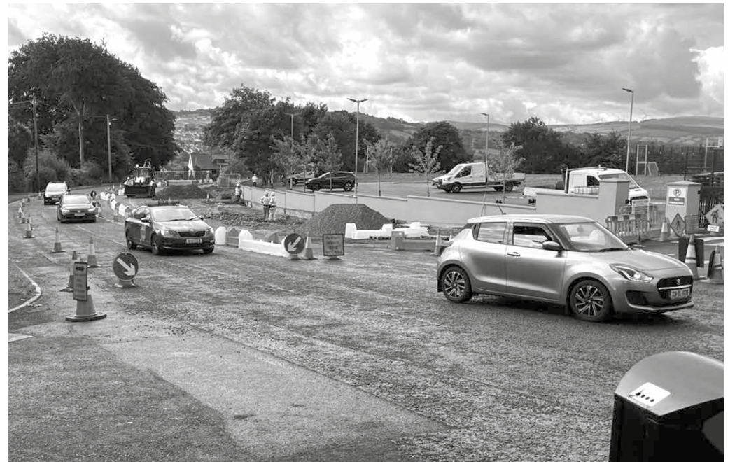
Works in progress at Convent Road in Letterkenny.
