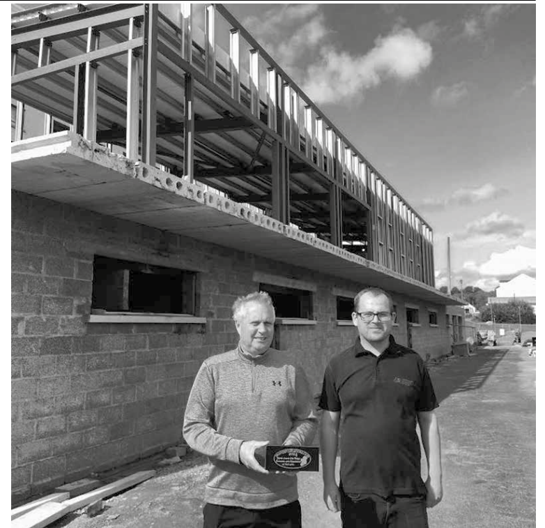
Liam O'Donnell, manager, and Lewis Toye, staff member, Letterkenny Community Centre, with one of the bricks which are part of the buy-a-brick fundraising campaign for the new Jim Lynch Community Building which is currently under construction.
