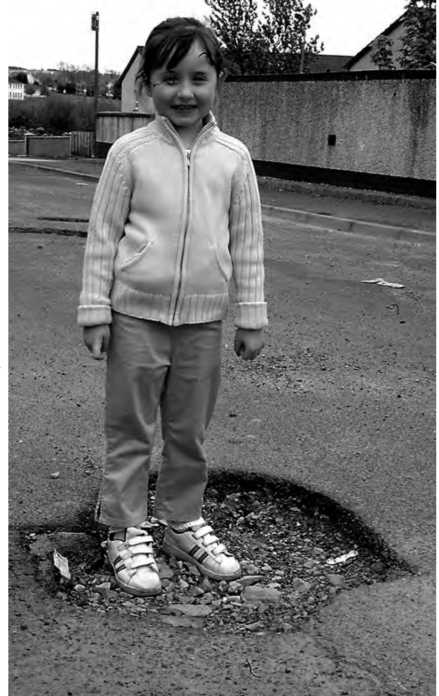
7 year old Kealey McDaid among the potholes in Meadowbank.
