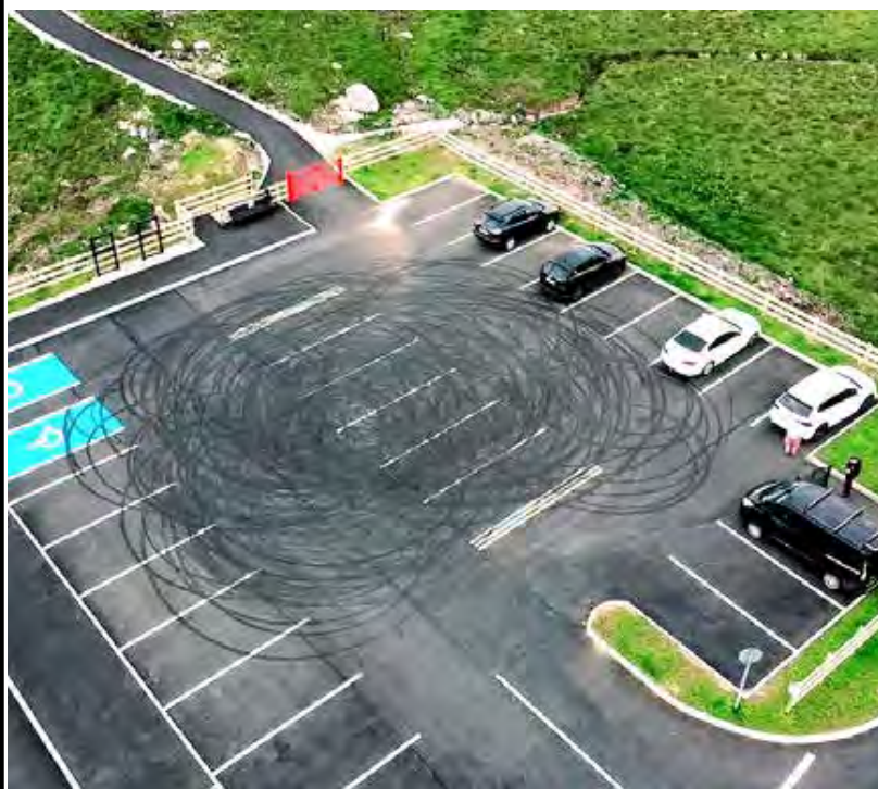
Damage at the newly completed car park.
