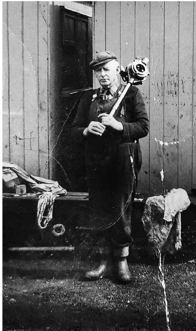
Willie McBride from Milford pictured carrying a pipe threader at work as a pipe fitter with William Press in Glasgow circa 1970. (Image courtesy of Sheila Friel)
