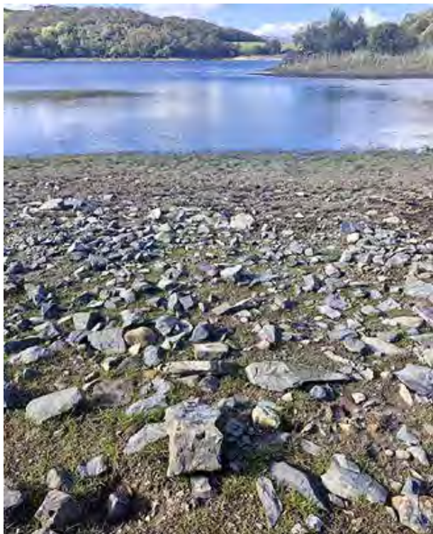
The Lough bed that should have 3m of water.
